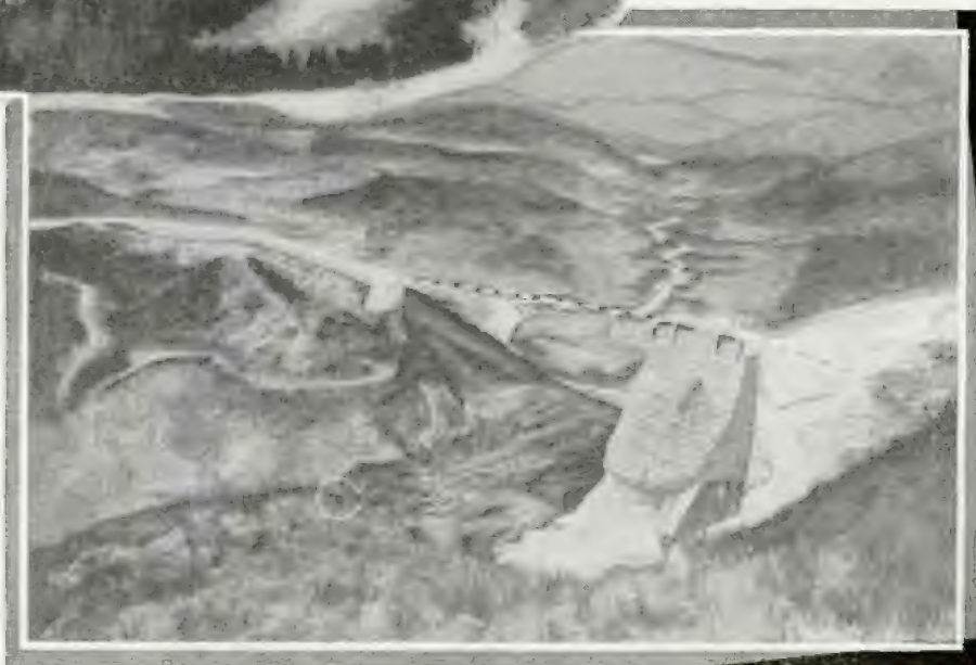
St. Francis Dam, after it had burst; note that the center portion still stands in place. Huge size of dam may be judged by noting man in white circle. Dotted line shows original dam contour.
