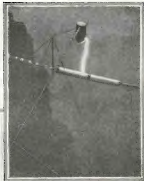
Actual photo above shows 13 ft. heavy spark obtained from the collecting net in the Alps by the German scientists. The voltage is about 2,000,000. The spark occurred once per second for 30 minutes.
