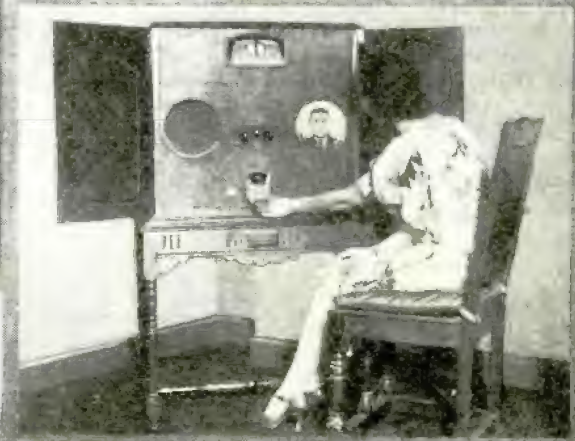
Photo at right shows the Baird experimental television receiver for both voice and image. The loud speaker is at the left, while the lens and its television image are seen at the right. The receiver is shown in the act of tuning in a station.
