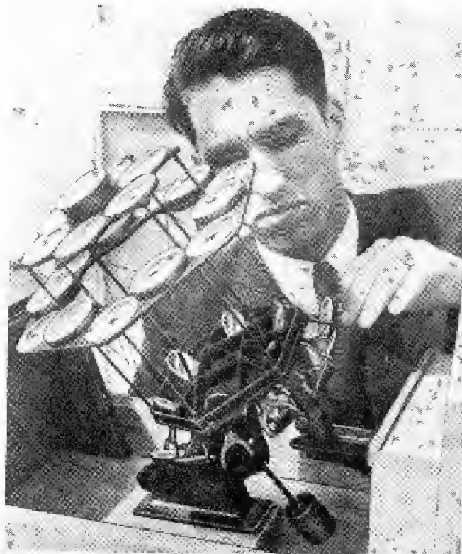
A model of a solar furnace which may melt diamonds, built by scientists of the California Institute of Technology, Pasadena. Each of the 19 lenses sends its ray to a common focal point at the base of the instrument. Below—An experimental sun engine using sulphuric ether as the working fluid.
